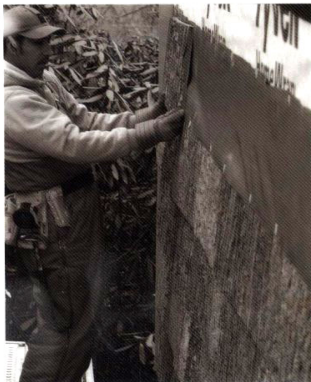
José installing poplar bark siding
