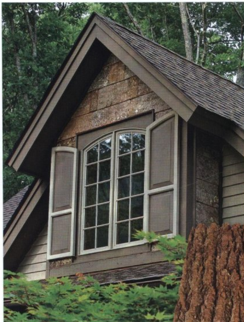
Poplar bark siding was used in the past by landowners who wanted to sell chestnut trees on their land instead of use them; now with chestnut trees destroyed by blight, poplar bark adds the rustic touch to today's mountain homes.
