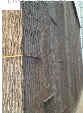
Exterior Bark Panels installed on a floating home.
