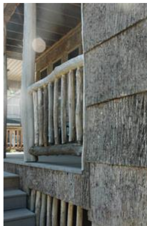
A bark away: The standard criteria for selecting siding typically concerns cost, durability and design. A few additional issues to consider when building green and with sustainability in mind: resource efficiency, embodied energy and performance. photo courtesy of Highland Craftsmen Inc./Barkhouse
