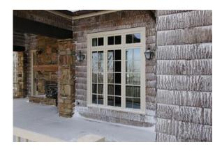
Thinking about re-siding your home? Take a look at this eco alternative. Just like a trees own weather proofing, these bark shingles insulate, protect, and are virtually maintenance free. It is made up of tulip tree bark waste from timber operations that would otherwise get burned, mulched, or left to rot.
