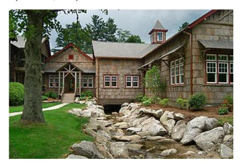
This is just too cool not to post. It's the bark of the poplar tree, harvested by hand when a tree is cut down. The bark is then flattened, dried in a kiln, then graded for thickness. It is then sold as siding for your home.
