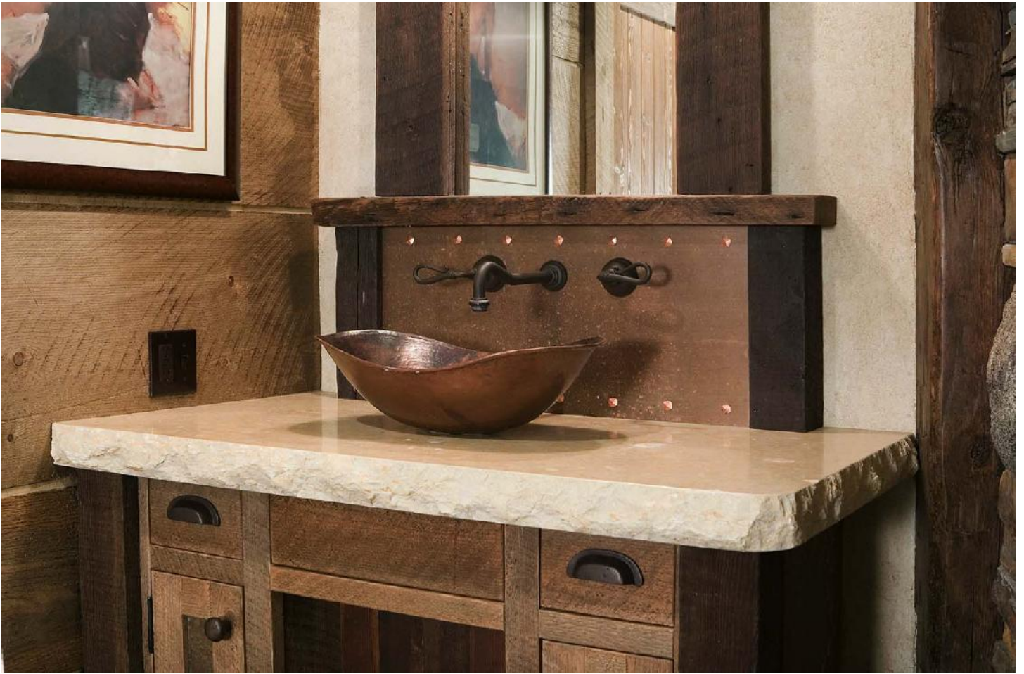
Above: The backsplash is sheet metal that has been antiqued with copper rivets. The wood used for the vanity is Dead Standing Pine which is reclaimed-resawn. On the vanity is Watco Medium Walnut stain. For the door inserts – Watco Dark Walnut Stain. The countertop is travertine with a 3" cracked edge detail.
