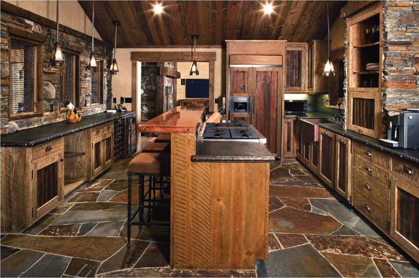
Above: The counter material is black honed granite. For added interest, a custom hand-forged ornate iron trim with copper rivets were added as a cap around the edge of the counters. The metal work was done by a Local blacksmith artisan in Tahoe, California. The flooring is random pattern flagstone slate.
