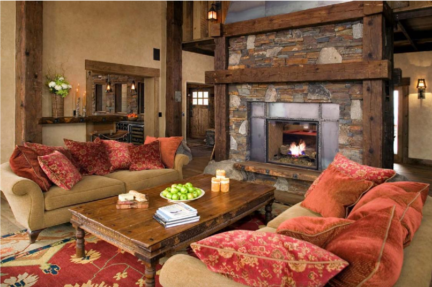
Above: The fireplace of this rustic mountain retreat features a solid stone. Its a combination of slate flagstone, slab, and stacked stone, incorporating reclaimed timbers and a sheet metal two sided fireplace insert. Its a tremendous focal point in the room as well as a great heat source.
