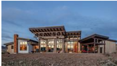
This Home Has Rusted Roots
