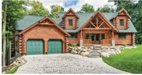
Coming Together at this Wisconsin Hybrid Home
